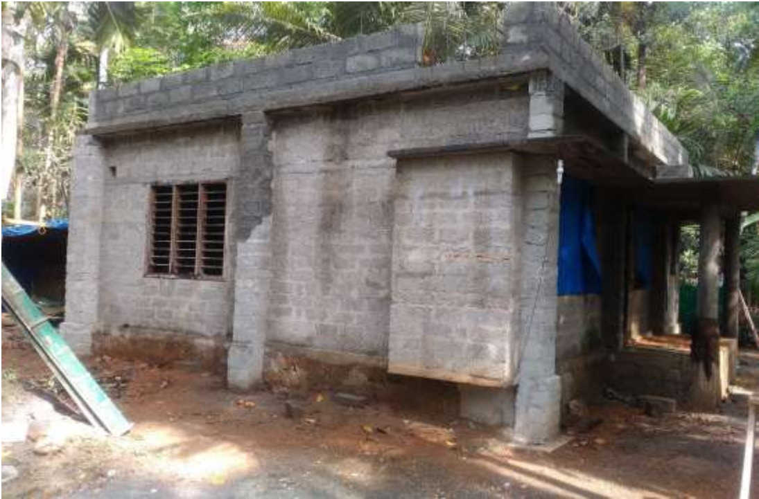
Different stages of renovation works
